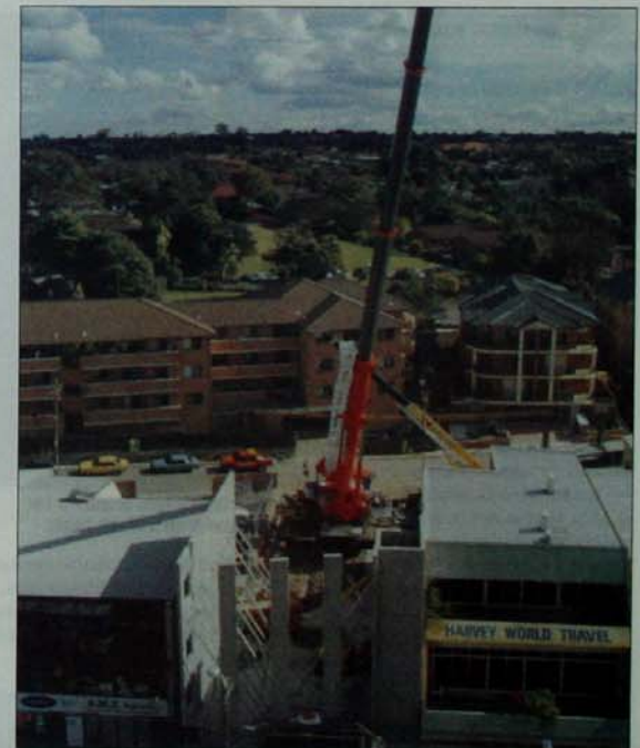
Aerial view of wall panel erection at narrow Rockdale site.
