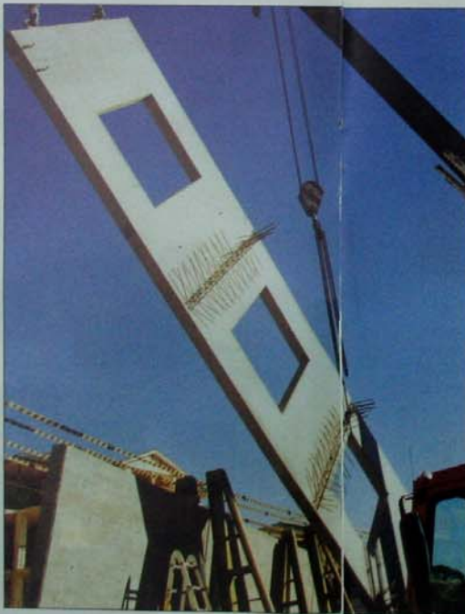
Lifting and turning 3-storey high (9.8m long) wall panel into position
