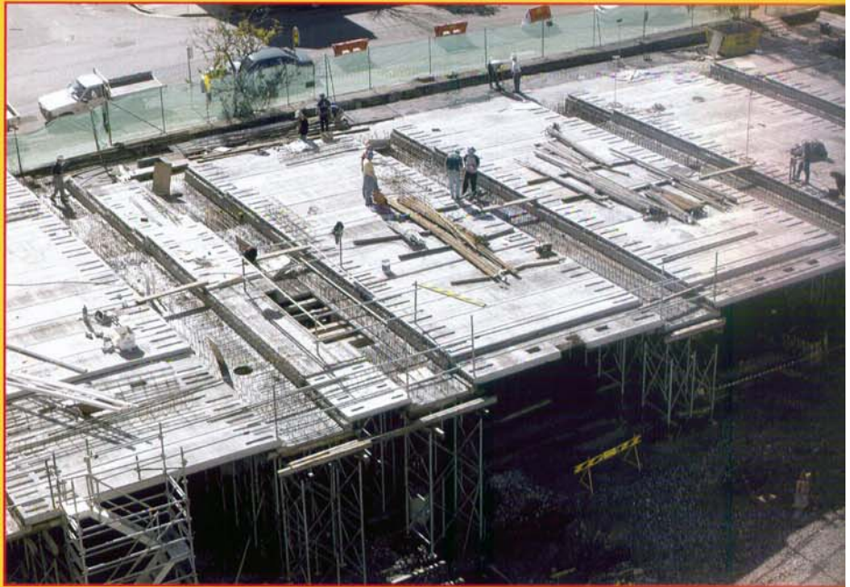
Hollowcore planks span between 2000mm-wide beamshells to form the transfer podium.
